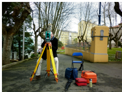
Fig. 19 – Total station used for the topographical survey
